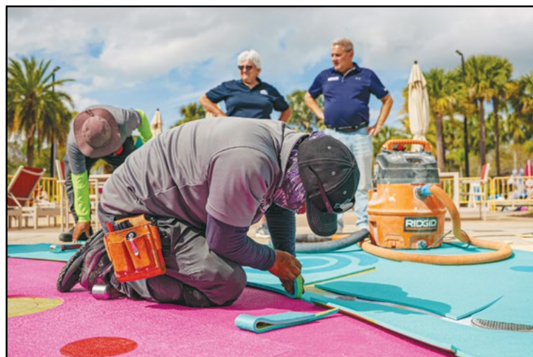
The Baynum team installed the Life Floor product at Give Kids The World Village. COURTESY BAYNUM
